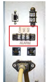
Remote alarm interface.
