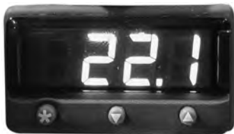
Temperature monitor/controller display and buttons.
