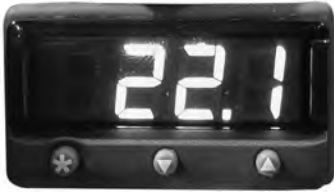
Temperature monitor/controller display and buttons.
