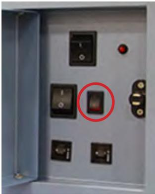
*i.C<sup>3</sup> Monitoring System / Access Control backup battery ON/OFF switch (circled)*
