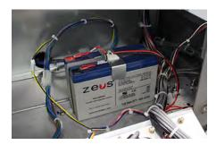
Monitoring system / Access control back-up battery
