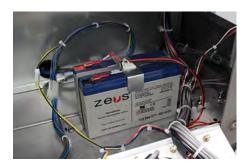
Monitoring system / Access control back-up battery
