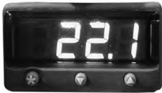
Temperature controller display.
