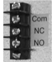
Remote alarm interface.
