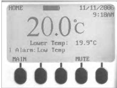
i.Center monitoring system.
