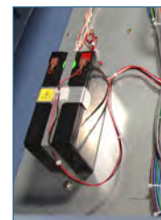
Monitoring system backup battery.
