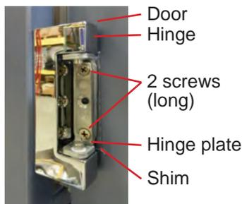
Hinge installation to door (lower hinge shown).
