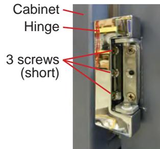
Hinge installation to cabinet (lower hinge shown).
