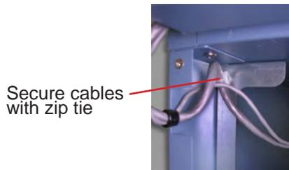
Power and communication cable(s) secured at hinge-side of the cabinet after hinge reversal.
