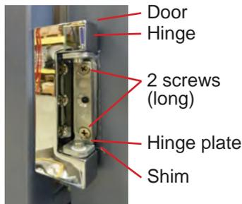
Hinge installation to door (lower hinge shown).
