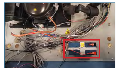
Monitoring system back-up battery.
