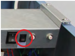
Figure 18 (left): Monitoring system / Access Control backup battery switch (circled). Figure 19 (right): Exterior door lock.
