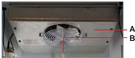
Drain line and hose.
