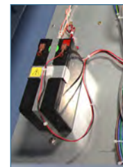
Monitoring system backup battery.
