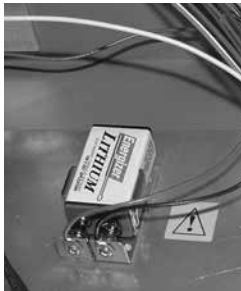
Monitoring system backup battery.
