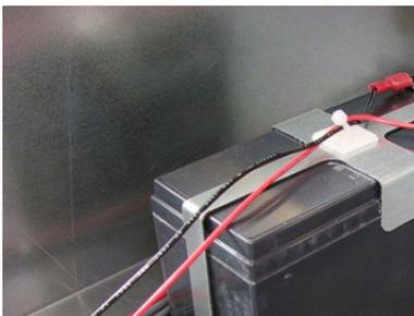
*Monitoring system back-up battery (supplies power to optional Access Control system).*
