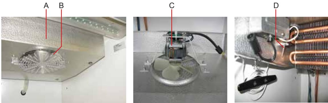
*Left: Unit cooler with fan guard. Middle: Unit cooler fan. Right: Temperature control probe.*
