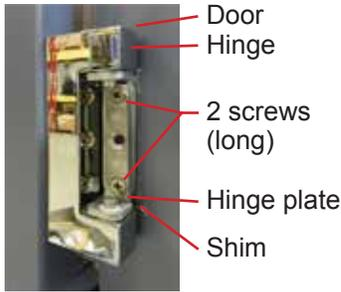
Attach hinge to door (lower hinge shown).
