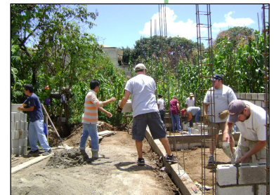
Guatemalan foreman assists Helmer team lay concrete blocks walls.
